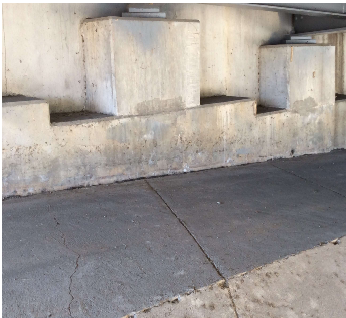
PHOTO 1 Description Bent # 1 vertical and horizontal cracking.
