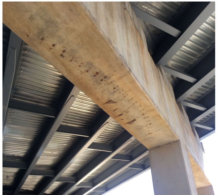
PHOTO 2 Description Bent # 3 spalling on the undersurface of the bent cap that exposes reinforcing steel with active corrosion.
